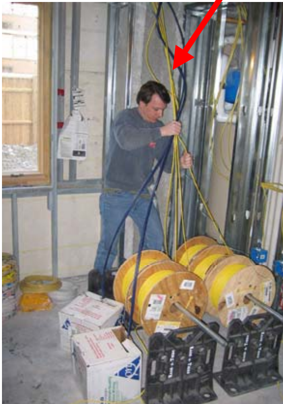
Figure 2 – Installation of Structured Cabling
